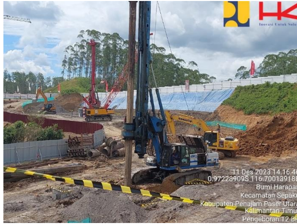
Gambar 70. Monitoring Pengeboran Pondasi Tower (Foto : Fabianty Edgar, 2023)
